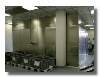
cleanliness is achieved at operator's breathing height. A physical barrier like pvc strip curtain or stainless steel walls, separate the booth from the external environment.
