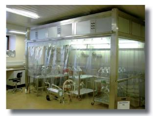
The Faster modules can be variously assembled together to build-up small to room size clean work areas.
